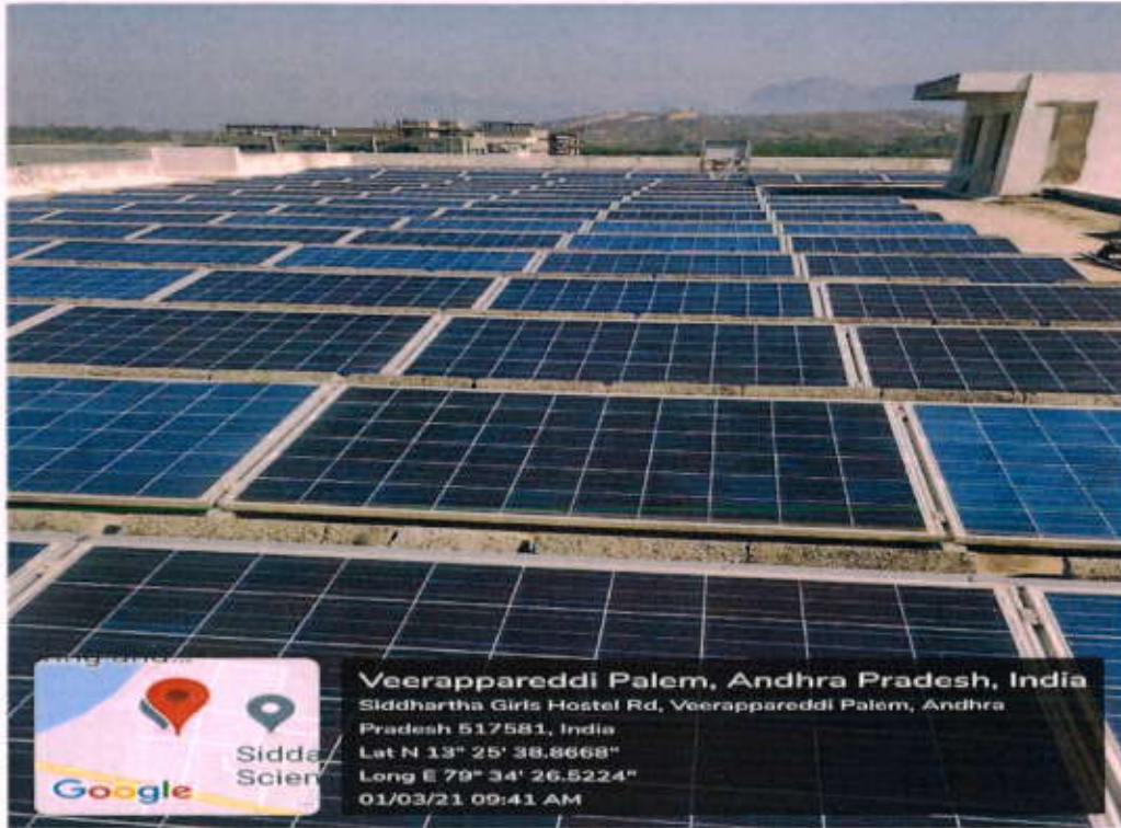
Rooftop Solar panels installed in the campus
