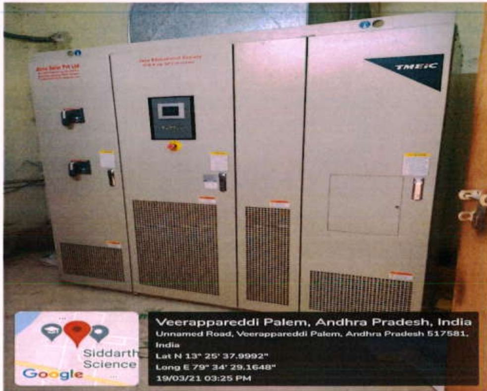
SOLAR PANEL BOARDS
