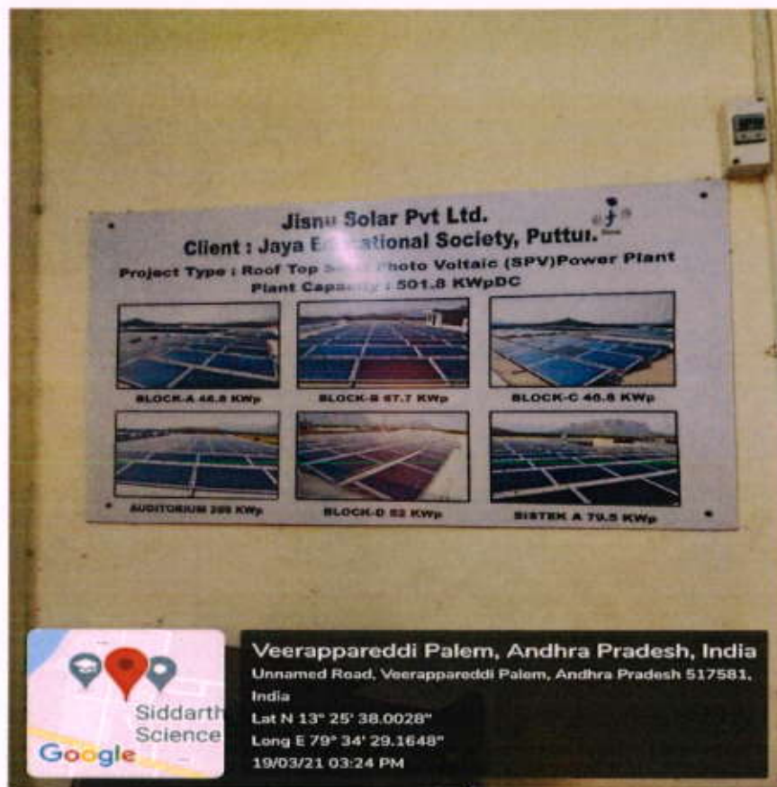
Rooftop Solar Panels Photos
