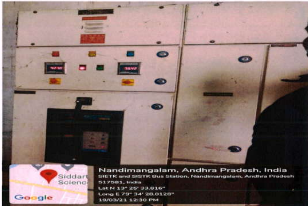
SOLAR PANEL BOARDS
