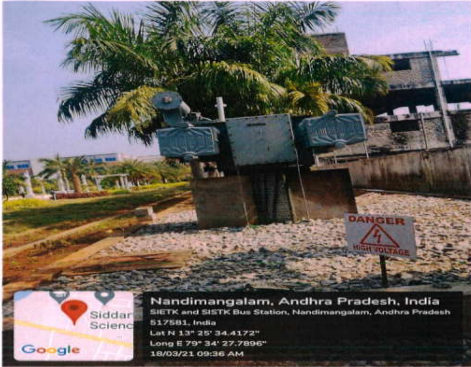
630kVA &500kVA Transformer installed in the campus (Energy Sourcefrom Southern Power Distribution Company of Andhra Pradesh Ltd. (SPDCTL)
