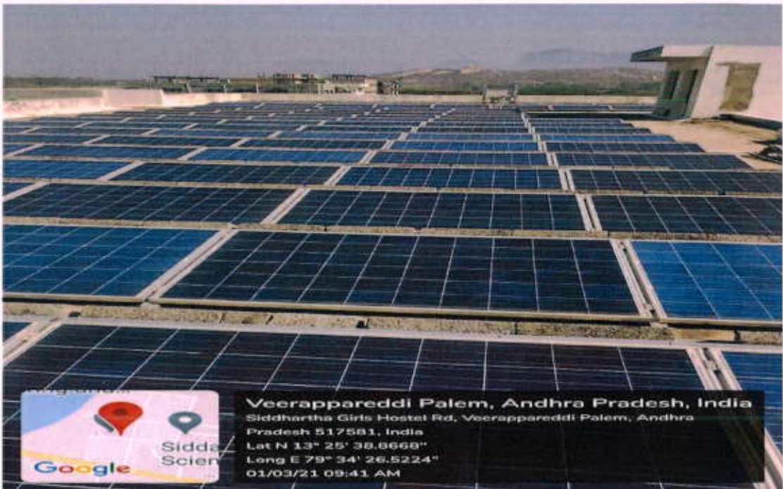
Rooftop Solar panels installed in the campus
